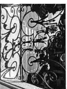
Garde-corps - APRES RESTAURATION - RCE
